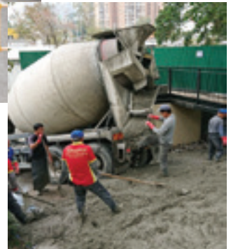
Re-cast new concrete slab 150mm thick
