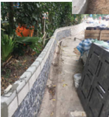
Rebuilt 650mm high planter curb
