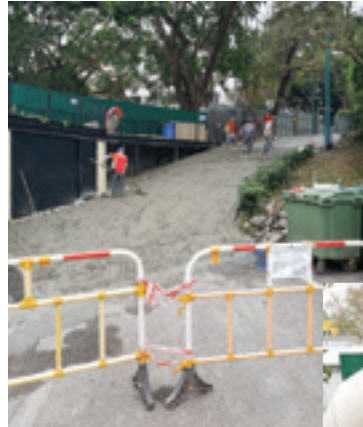
Re-cast new concrete slab 150mm thick
